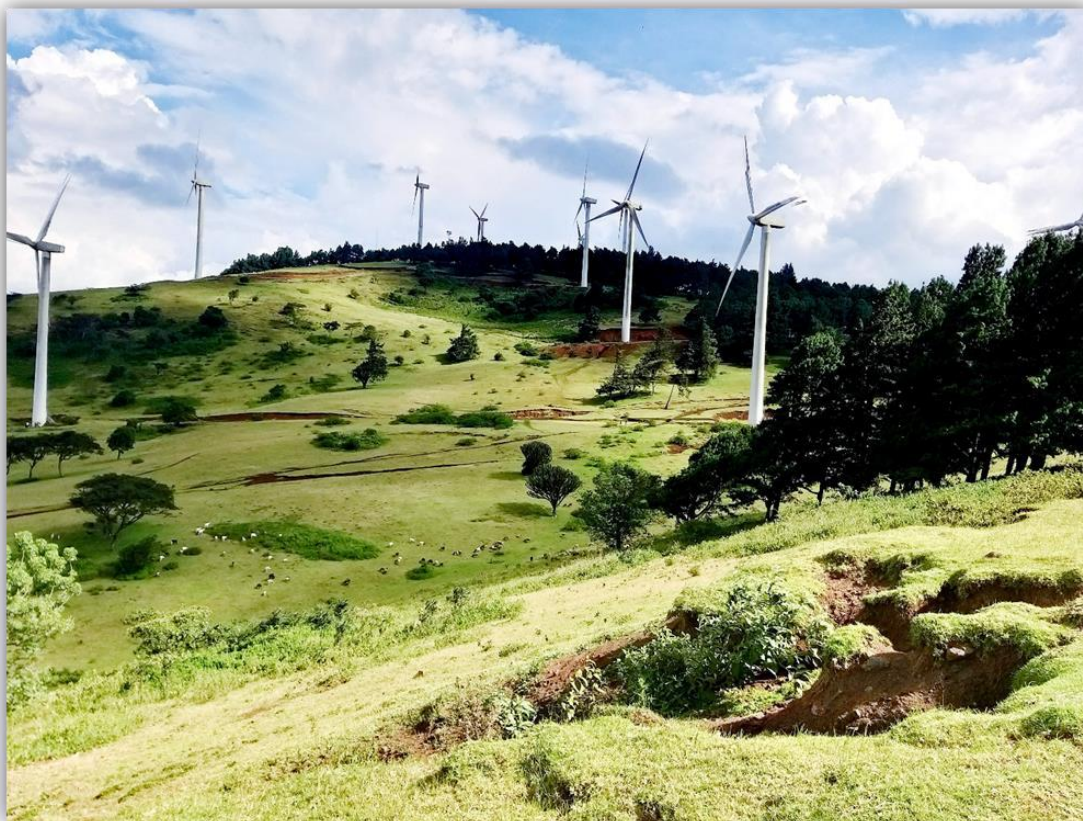
Figure 5-8: Ngong Wind Power Station in Kajiado County
